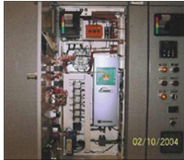
Motor Control Centers consists of six [6] Soft Start Starter buckets, six [6] Variable Frequency Drives [VFD's], and an Auto-sensory and Control section. Additionally there is modem/router to communicate with SCADA.
